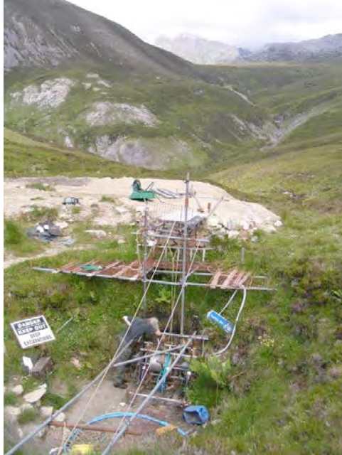
Figure 8 – Infrastructure to aid digging work within Rana Hole 2009.
