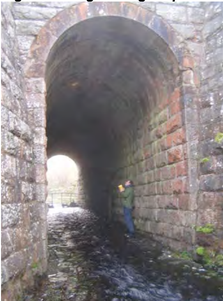
Fig. 2 – Bridge being inspected
